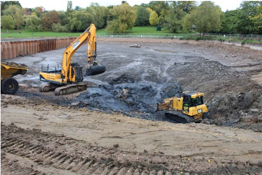
Picture 2 - De-silting Model Boating Pond using excavators
