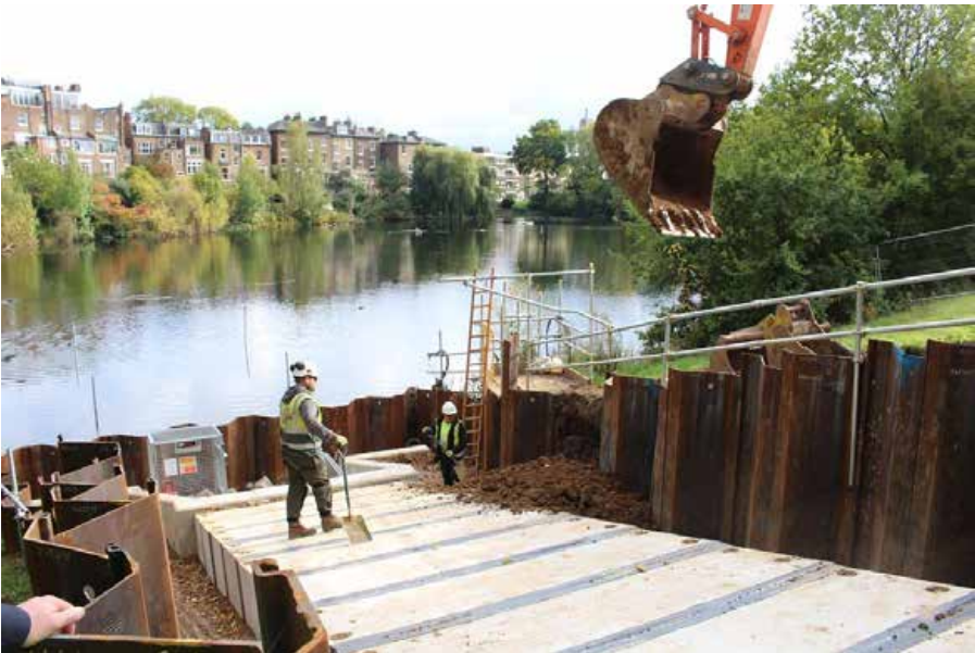
Picture 6 - Works underway building the culvert between Hampstead 2 and 1.
