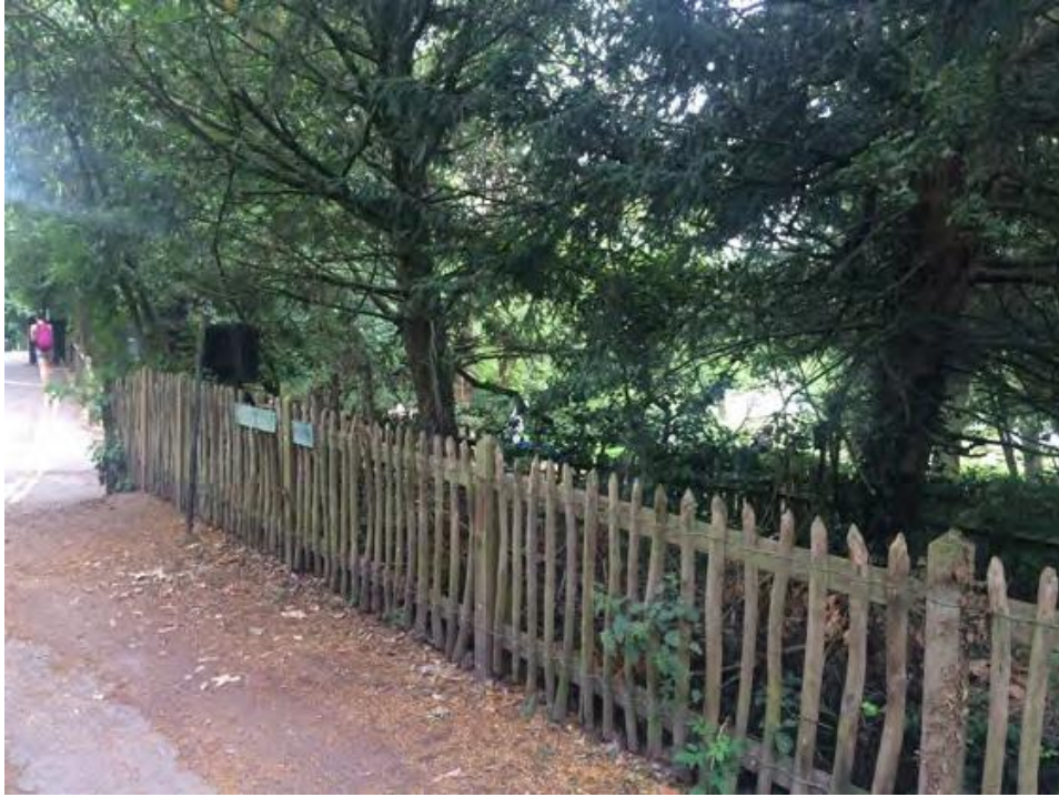
Figure 5 – Remove chestnut pale fencing and replace with timber post & rail (Note 6, appendix 3 - proposed layout)
